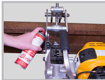
Drill the hole. Apply the cutting oil.
